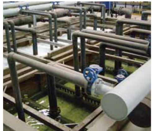
**Inner Mongolia** – KMS has installed its first-ever large-scale, ultrafiltration systems in China.
