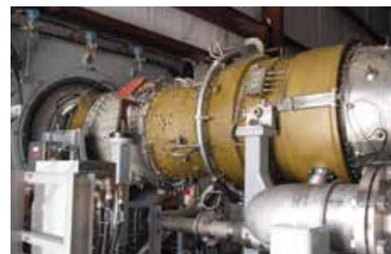
This Rolls Royce jet engine is one of five that supply regeneration air to the plant's reactors.
